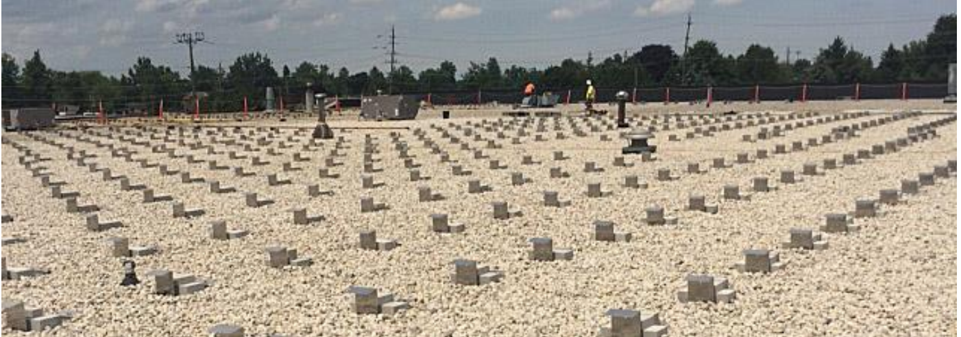
360 kW DC FIT 3.1 Project located in Orangeville, Ontario currently under construction.
