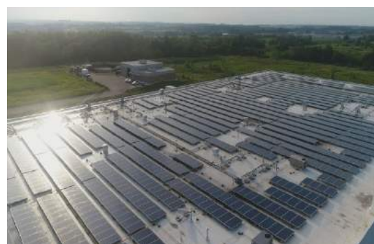
600 kW DC FIT 2 Project located in Ajax, Ontario, completed in October 2015.
